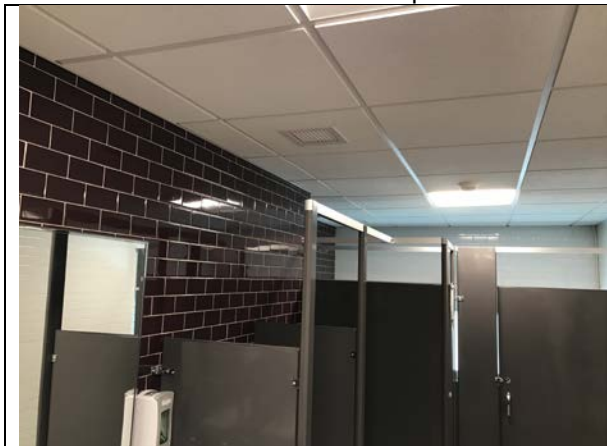
New Boys Bathroom with Exhaust
