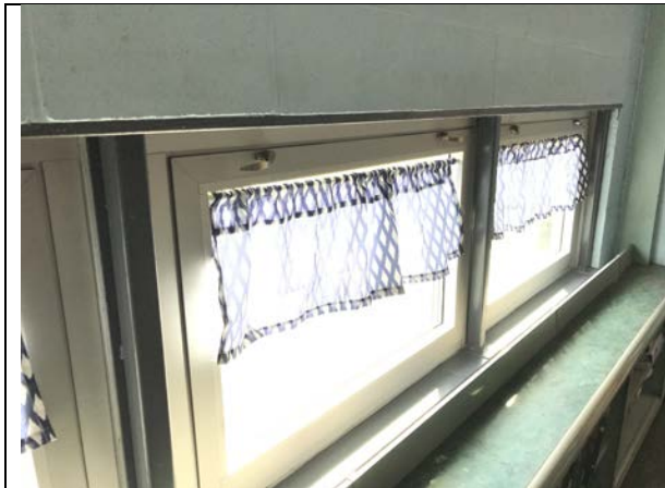
Classroom Operable Windows
