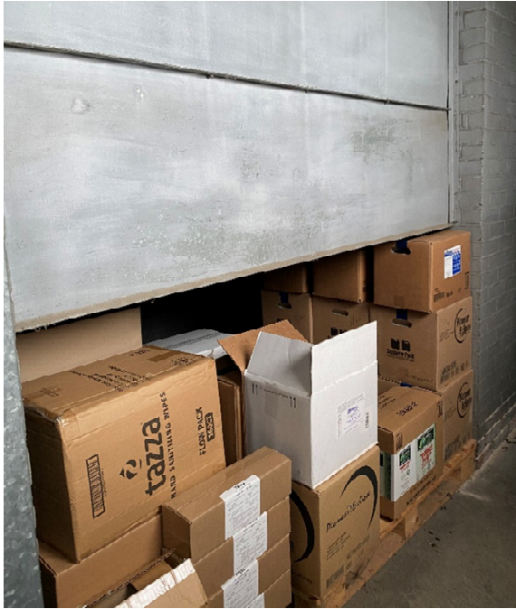
Picture #1 & 2: Typical obstructions to natural ventilation system
