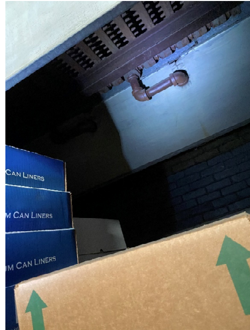
Picture #1 & 2: Typical obstructions to natural ventilation system
