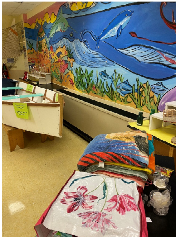
Picture #1: Classroom with sill mounted Unit Ventilator
