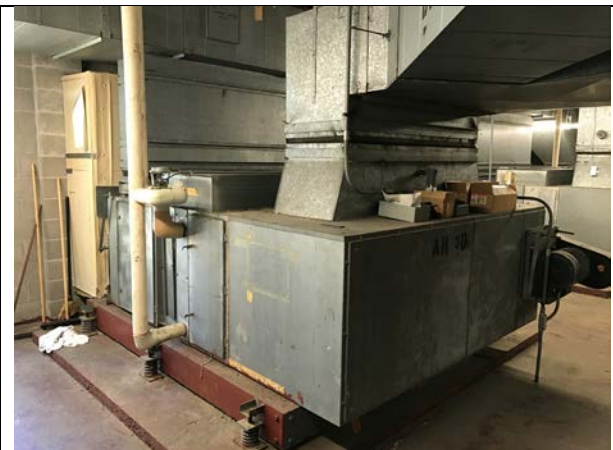
AH-3D (Boys Locker-room)
