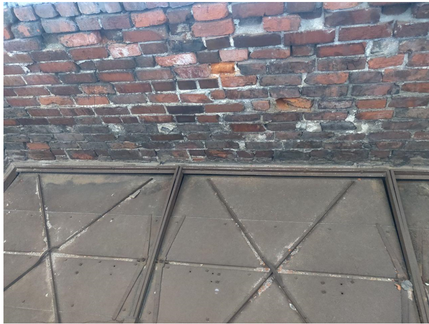
Picture #9: Photo taken of inside Natural Ventilation Shaft on Roof.
