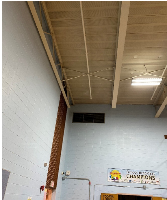
Picture #3: Auditorium / Café Supply Grille
