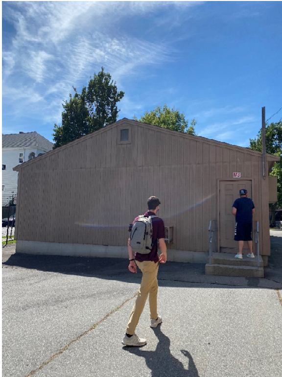
Picture #15: Modular Classrooms
