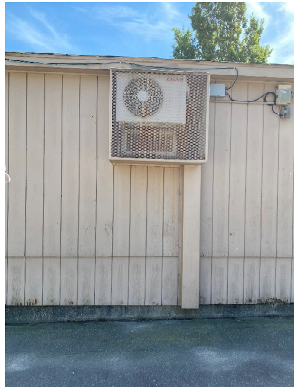
Picture #16: Modular Classrooms
