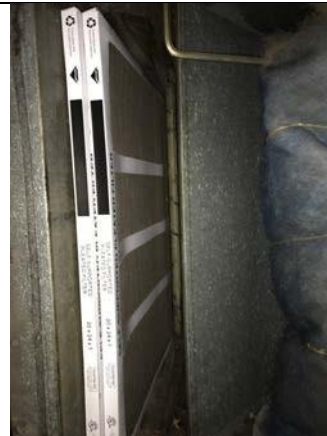
HV Filter and Internals
